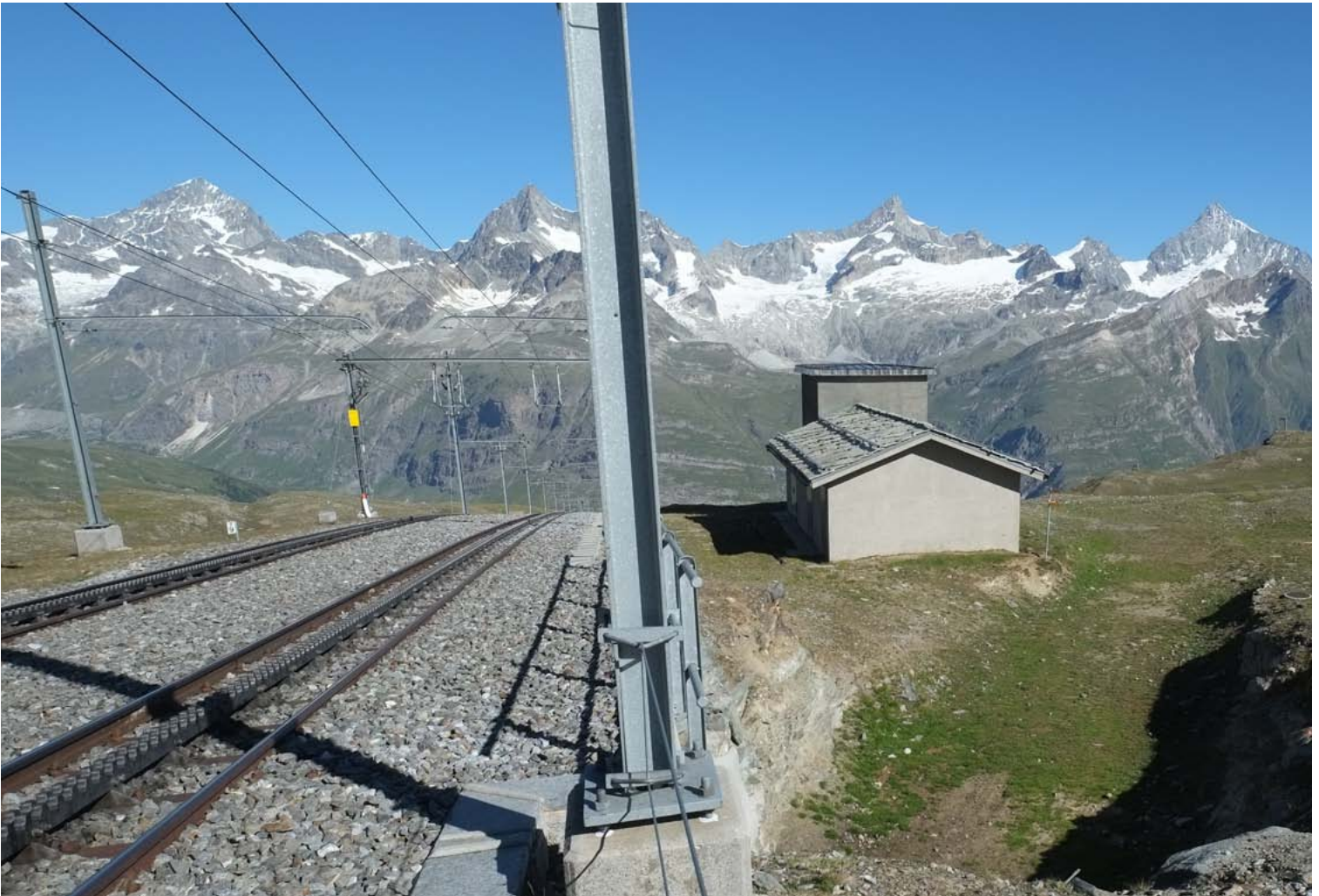
The rack rail is visible in this image of the Gornergrat line disappearing down the hillside, with magnificent panorama views of the surrounding mountain ranges. Photo: architecum 2018
